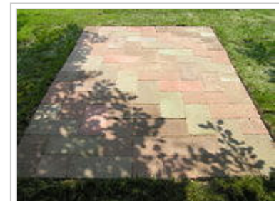
Concrete paver blocks laid in a rectangular pattern
