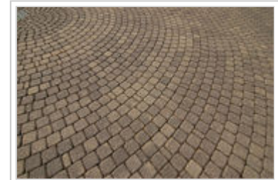
Concrete paver blocks laid in a circular pattern
