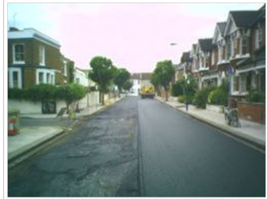
A road in the process of being resurfaced, showing both old and new asphalt surfaces.
